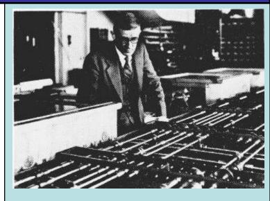
The original differential analyzer was a physical machine developed by Vannevar Bush at MIT in the 1930's in order to solve ordinary differential equations.
